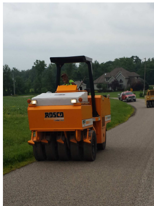
Count Forces chip and seal county roadways.
