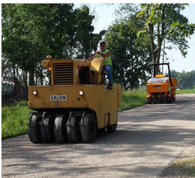
Count Forces chip and seal county roadways.
