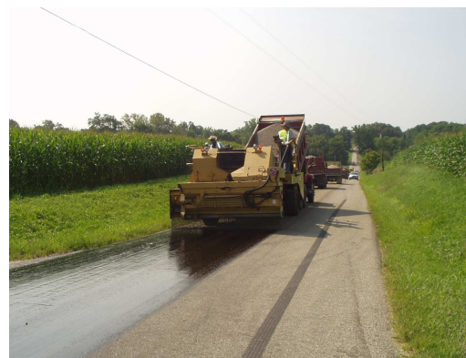
County Forces Chip & Seal (above)
