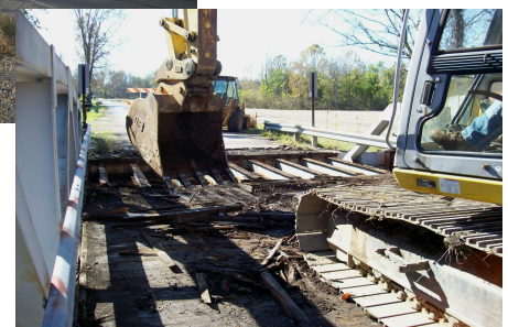
RIC-12 BRIDGE DECK REPLACEMENT (right)
