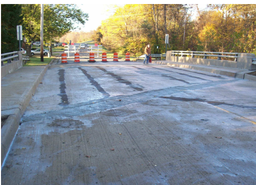
County forces perform a deck rehabilitation on the HOC-04 Bridge on Boving Road. (pictured above)
